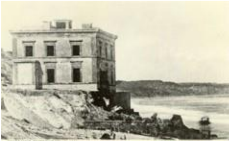
Figure 2.1 (left): 'Simpson's Folly' was built at the foot of Canford Cliffs near Bournemouth in 1878. Insufficient consideration was given to coastal erosion and the property had to be demolished soon after its occupation.
