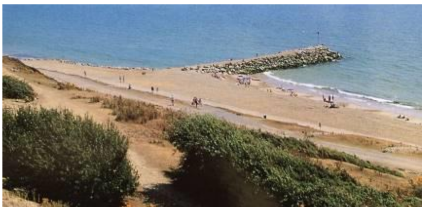
Figure 1.8: Highcliffe beach today. The rock breakwaters, beach replenishment and cliff works help to protect the frontage. The frontage has a 'Hold the Line' coastal protection policy for the next Century.
