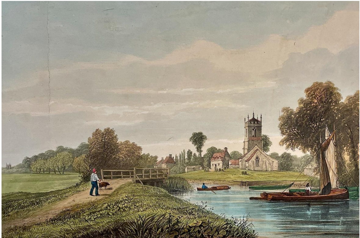
Figure 11.1: The hamlet of Hartford on the Ouse , a copperplate engraving. c.1830. This picturesque view shows the church close to the river bank which is now strengthened by a wall instead of timber breastwork. The river is wider and the jetty has gone but otherwise the scene has changed little. The wider floodplain can be seen on the left of the engraving. Figures 11.2 and 11.3 (below) show the vicinity today.
